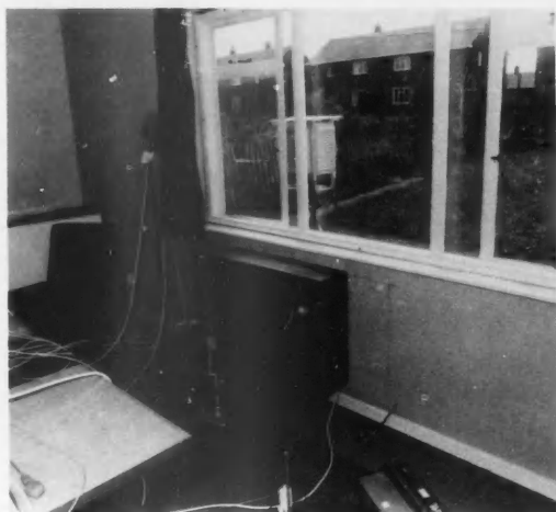
Fig 6 Indoor and outdoor views of a 2 kW air-to-air heat pump designed for single-room heating and installed in a trial house.
